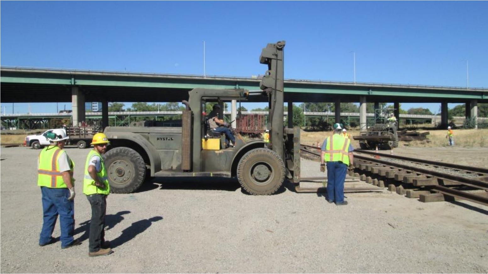
Simba and Big Green working in tandem: Leonard on Simba gets ready to move some track panels as Mike H. on Big Green distributes ties
