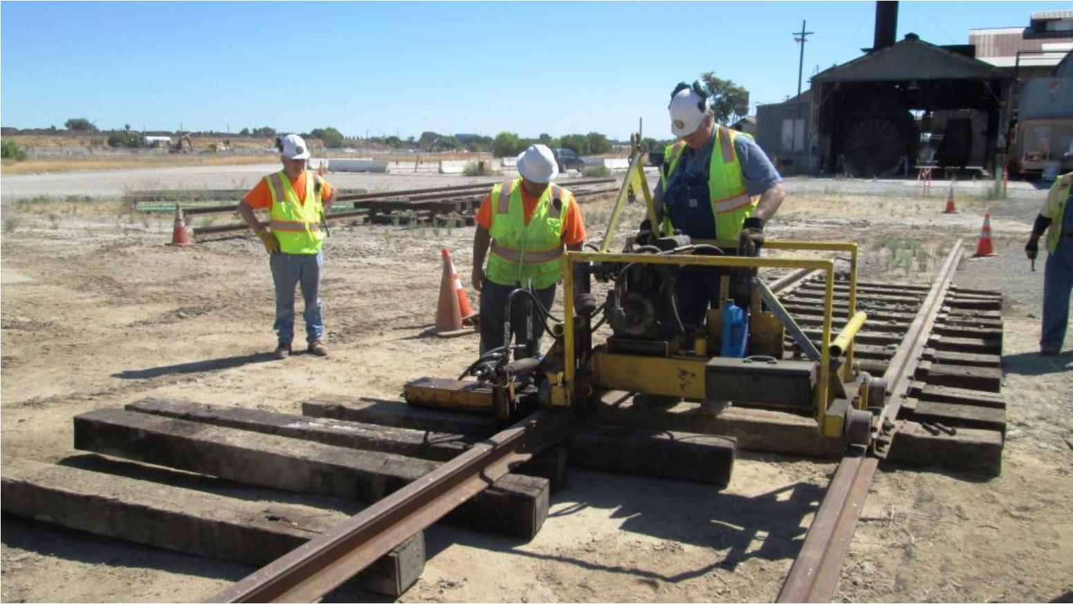
Anthony and Chris C. insert ties using the section-gang machine
