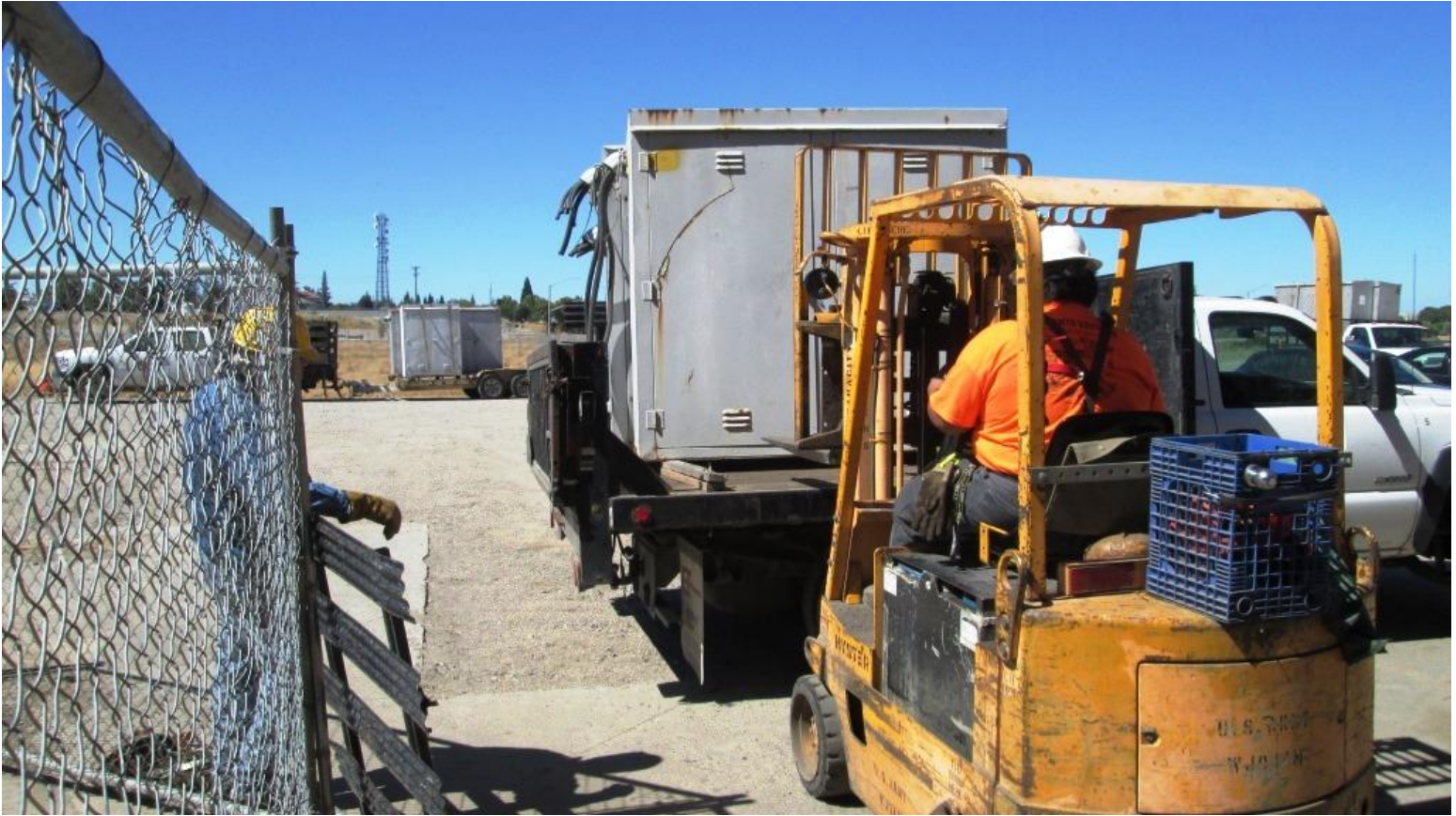
Anthony on the forklift unloads signal cabinets
