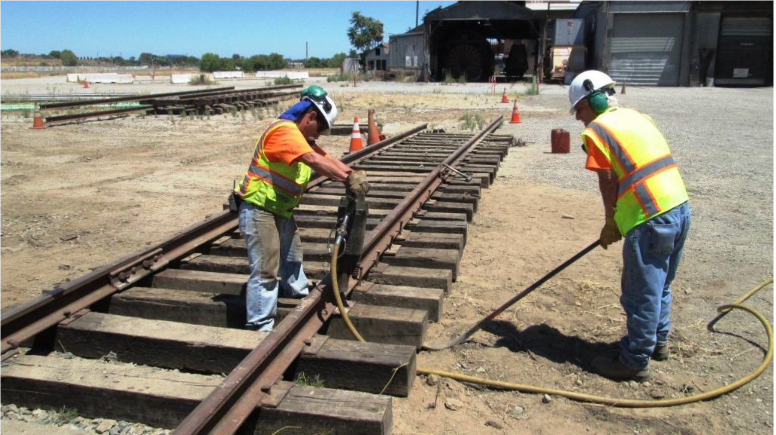
Back at it, Joe uses the 90-pound pneumatic spike drive to drive spikes while Mike W. nips-up the tie
