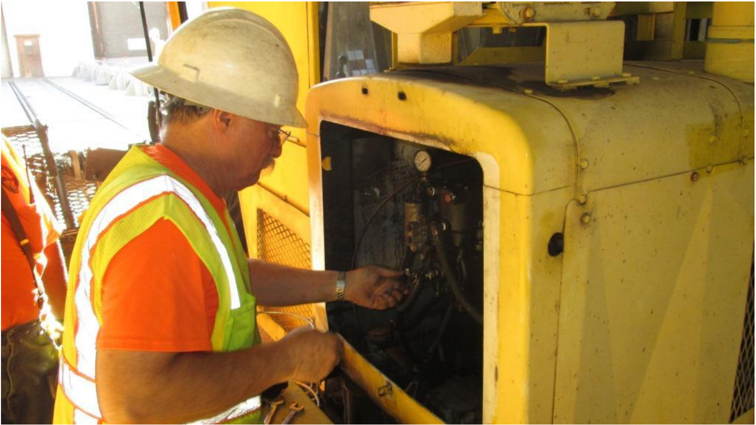
Mike H. makes a final check on the scarifier's new air-compressor
