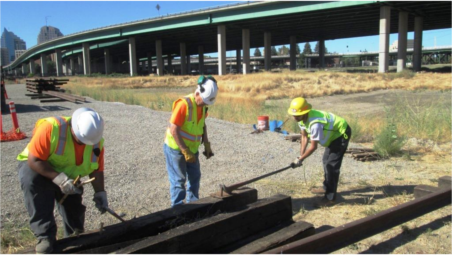
Anthony plugs spike-holes in the tie as Mike W. gets ready to grab the spike that Chris M. is pulling
