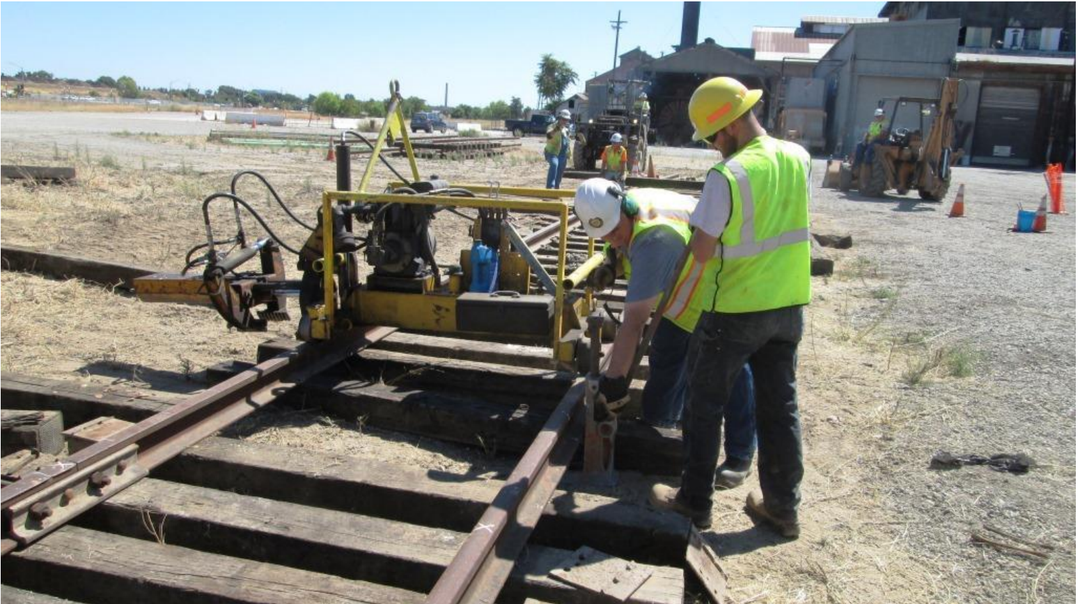
Chris C. and Chris M. use a track-jack to lift the rail so that the section-gang machine can slide a tie underneath
