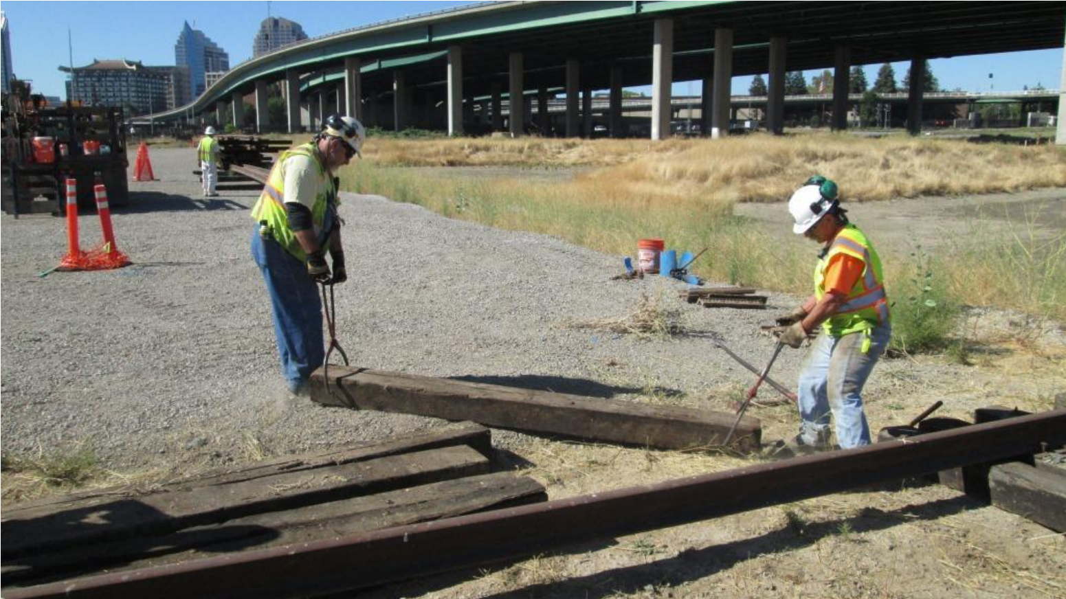
Mike F. and Joe move a tie into position
